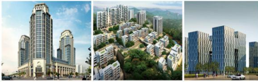
山东德州恒鸡美食城 Shandong Deyou Brand Chicken Delicacy City 山东海东佳苑 Shandong Haidong Residential Quarter 北京天元工业园 Beijing Tianyuan Industrial Zone
